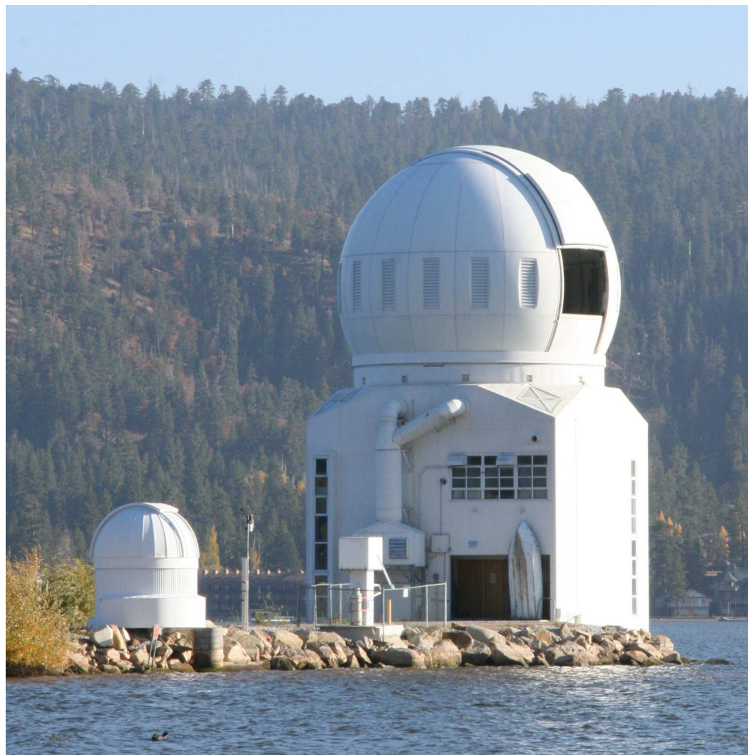
Big Bear Solar Observatory sits on the end of a 1000 foot causeway in Big Bear Lake, high in the San Bernardino Mountains of Southern California. In preparation for the 1.6-meter New Solar Telescope, the old, smaller hemispherical dome was replaced with a larger 5/8 sphere made of fiberglass. The small dome to the left houses the Earthshine and H \alpha full-disk telescopes.
